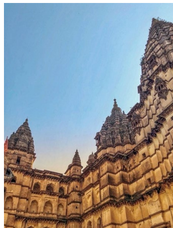
Figure 1. Chaturbhuj Temple’s splendid spherical spires 350 feet above ground level.
